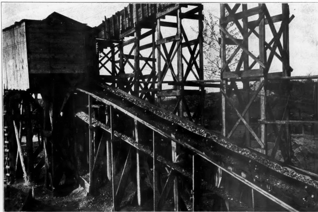
The Conveyor From the Tunnel to the Loading Bins
